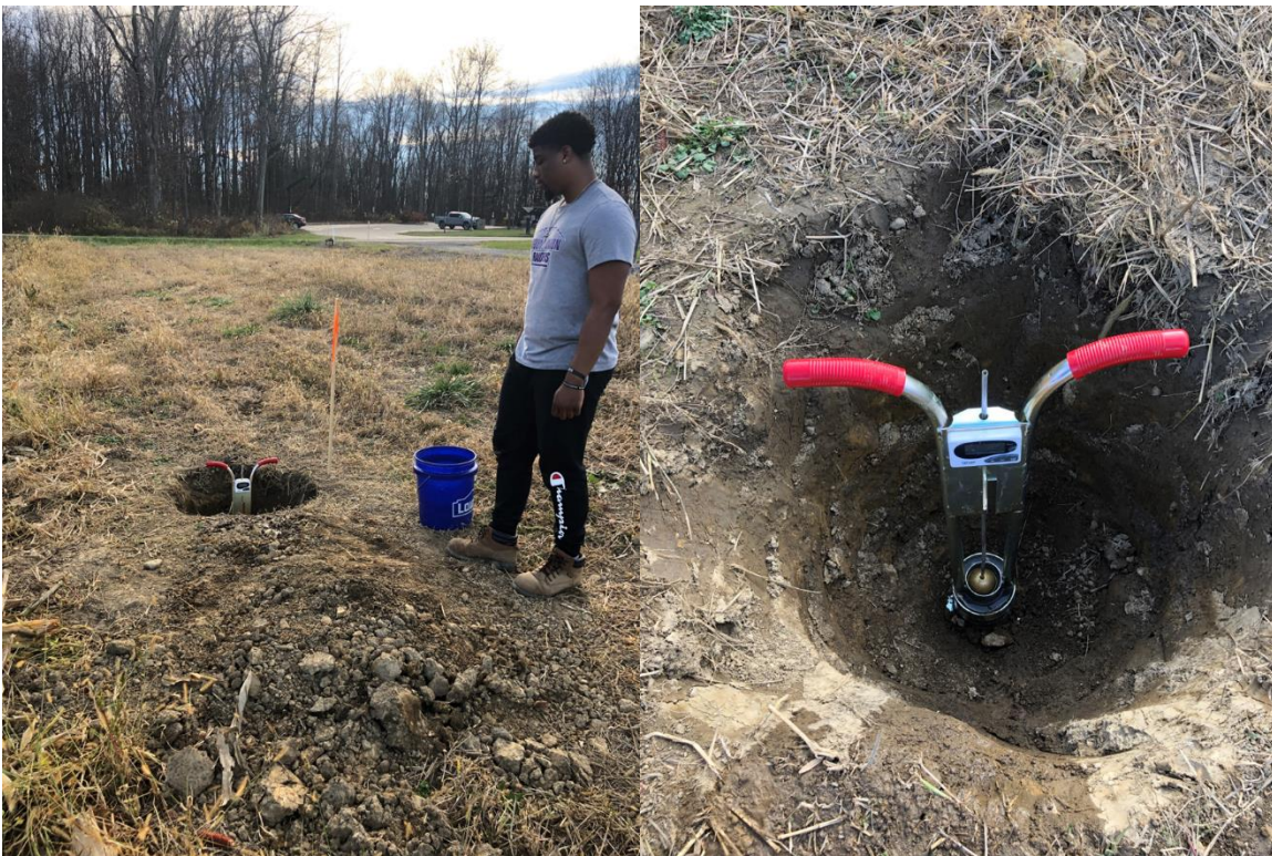
University of Mount Union civil engineering students (ECE 440: Sustainable Infrastructure Design) conduct infiltration tests at the surface and 1-meter depth with an infiltrometer to ensure the permeability of the soil is suitable for the creation of a wetland.
